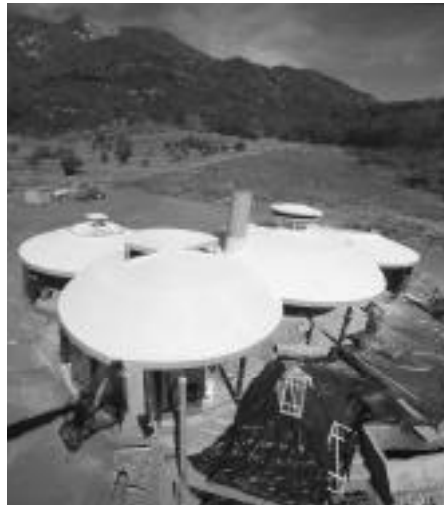
Finished roof of John Davis' home in Oak Glen, CA
